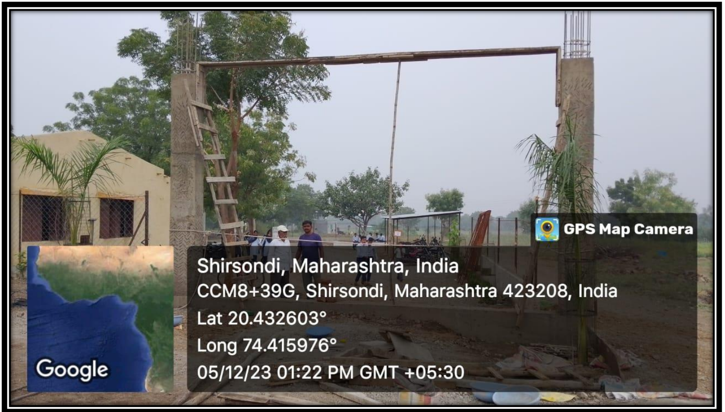
Work in Progress of College Entry Gate...
